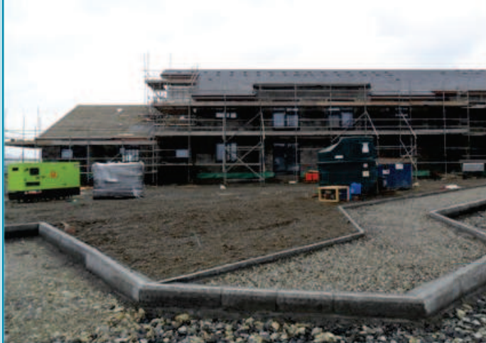
Mull Progressive Care Centre under construction
